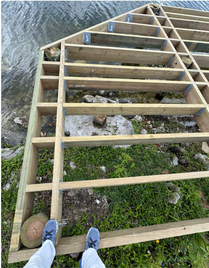
Figure 11: Peninsula Park Dock Framing/Piling System
