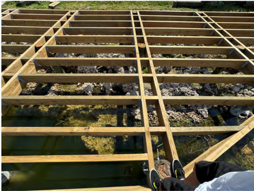
Figure 5: Clubhouse Dock Framing/Piling System
