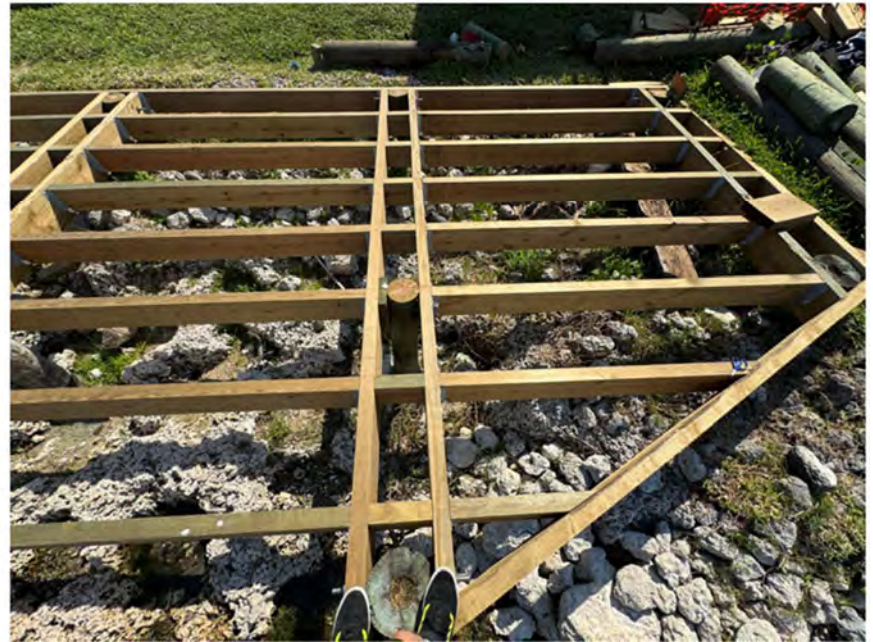
Figure 5: Clubhouse Dock Framing/Piling System
