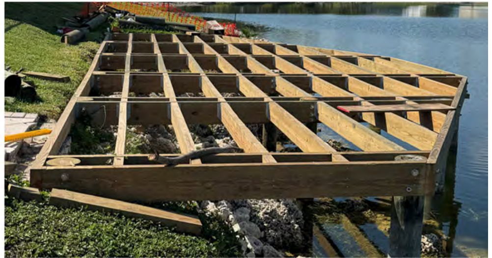
Figure 4: Clubhouse Dock Framing/Piling System
