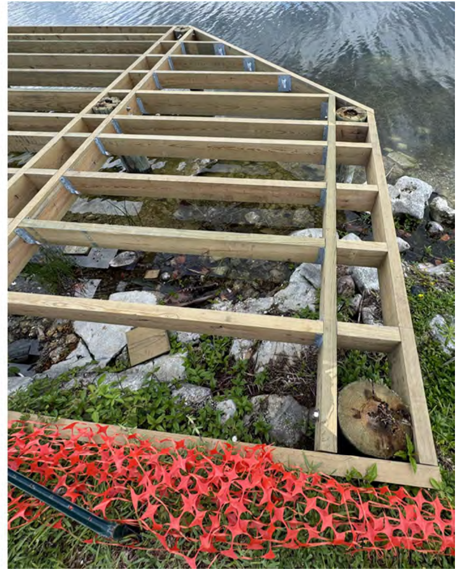
Figure 11: Peninsula Park Dock Framing/Piling System
