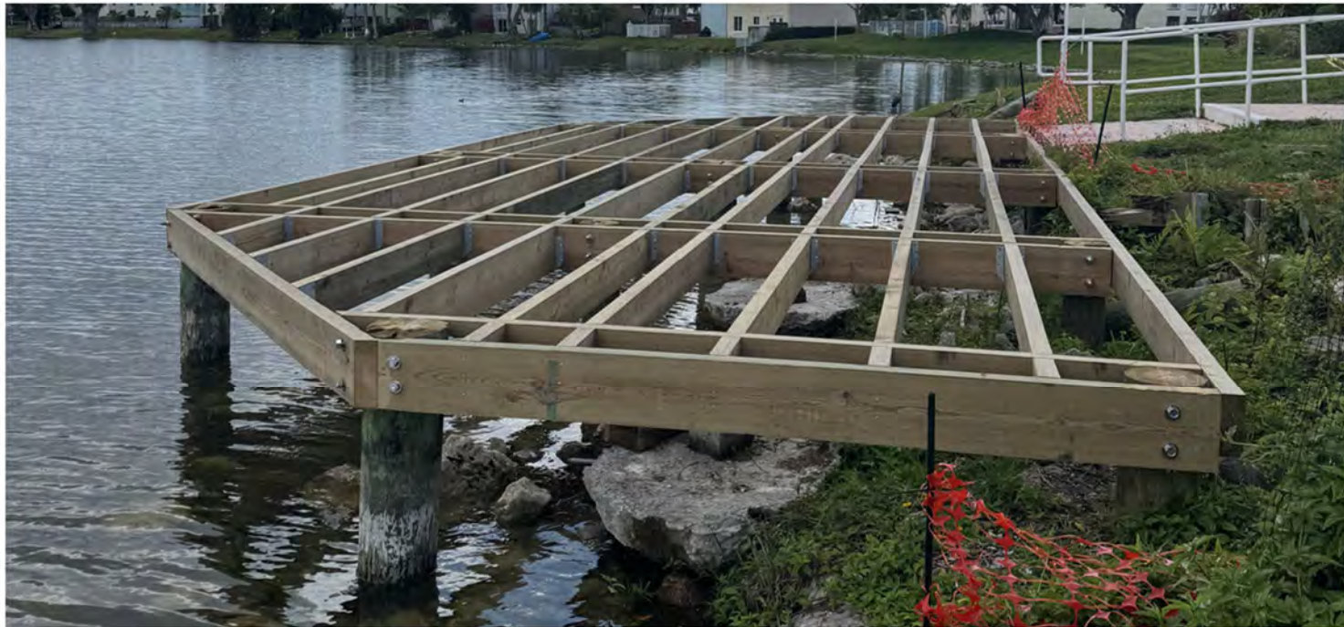
Figure 10: Peninsula Park Dock Framing/Piling System
