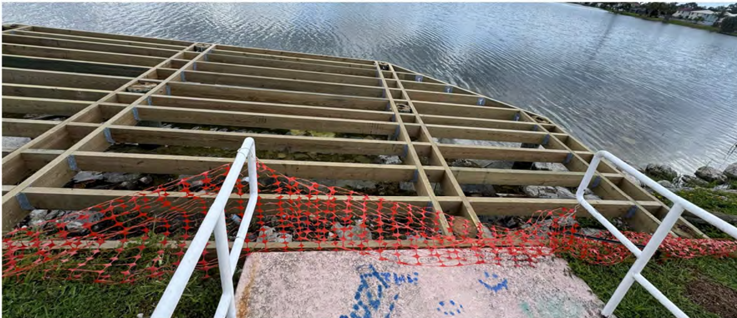
Figure 9: Peninsula Park Dock Framing/Piling System
